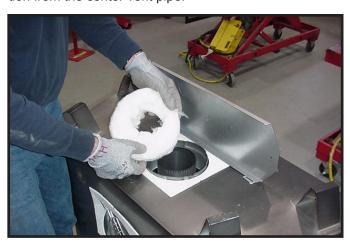
Figure 6.7 Remove the insulation from the outer vent pipe.
