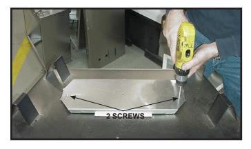
**Figure 6.2** For top vent, remove the two screws holding the top heat shield in place.
