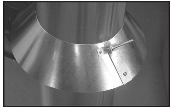
Figure 7.14 insert Bolt into Brackets
