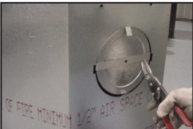
Figure 6.8 (Generic Appliance Shown) Cut the metal retaining band and fold the sides out.
