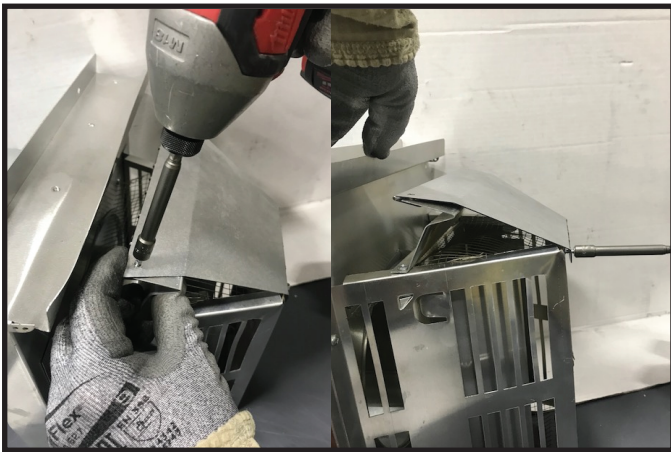
Figure 7.15 Wind Diverter Installed
