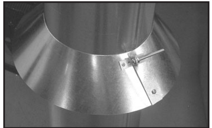
Figure 7.11 insert Bolt into Brackets
